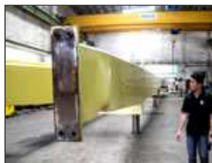
NMF slim line container crane boom repairs details...
