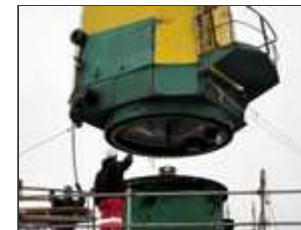
NMF crane removal and reinstallation from vessel details...
